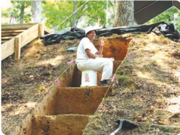
Types of excavation. Step trenching
